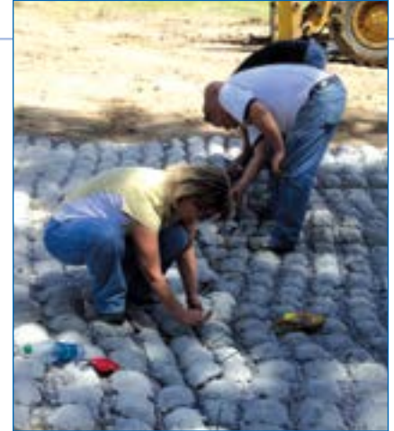
5 Inserting zip ties at seam.
