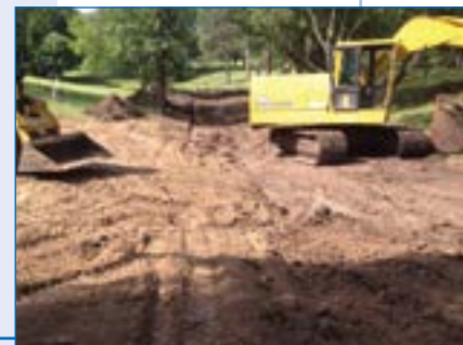
2 Preparatory dirt work.
