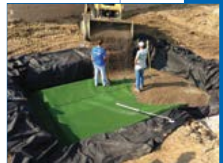
3 Micromesh separator still exposed as washed pea gravel placed on top.
