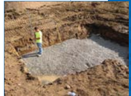
1 Gravel base in place and laser leveled.
