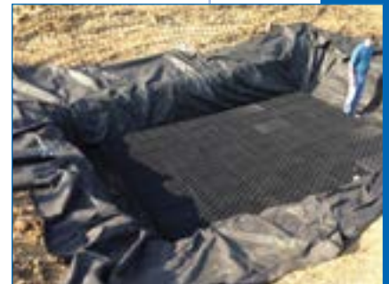
2 Atlantis Raintank underdrain installed to handle the high flow media.
