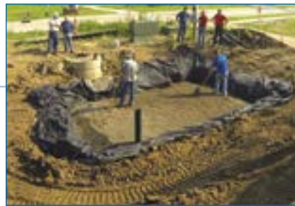
4 Final grading of the media is taking place before mulch installed.
