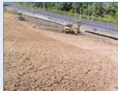
2 More grading of slope (prefer to have tracked equipment running up and down slope).
