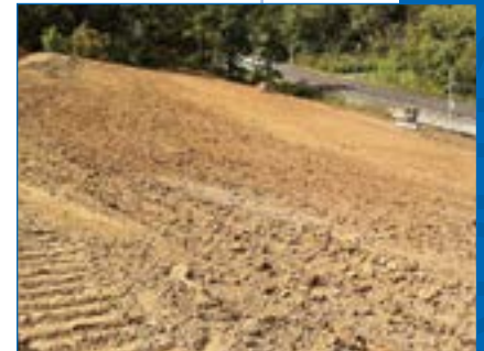
1 Grading of slope.
