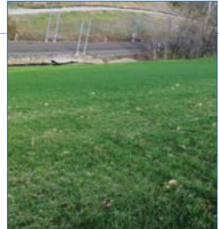
5 Another picture showing finished grading and vegetation establishment.
