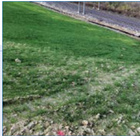
4 Notice the grading of slope (fine grade not necessary).
