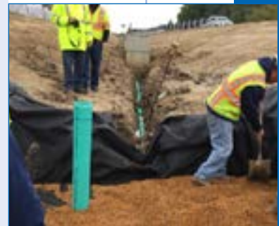
2 Miramesh TR and washed pea gravel.
