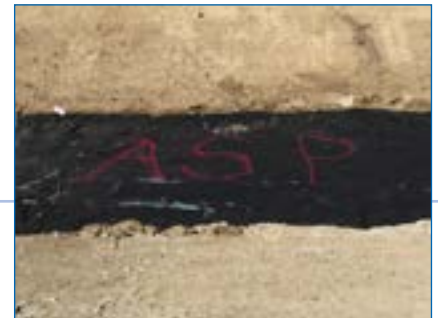
6 Buttoned-Up until Commissioning.
