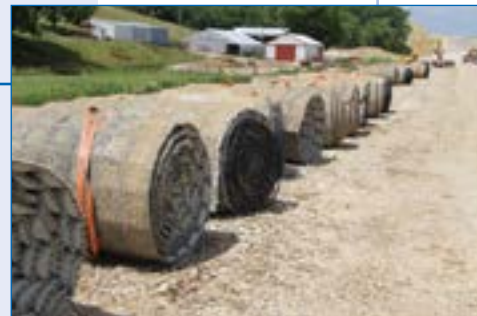
1 Flexamat Rolls off-loaded and staged along the channel.
