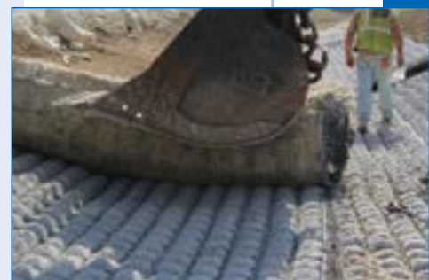
3 Flexamat rolls laid by nudging them with the track hoe bucket.
