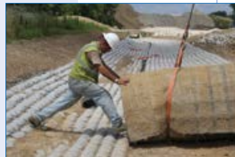
2 Flexamat installation with 1 track hoe operator and 1 worker in the channel.
