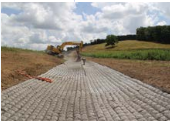
6 Final adjustments are made with the teeth on the bucket.
