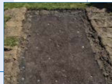
2 Repair failed areas to proposed grade, compact & place permanent TRM.
