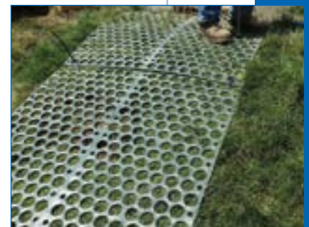
3 Anchor ScourStop with Bullet-Shaped Percussion Anchors.
