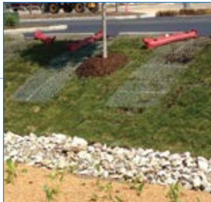
6 Completed ScourStop installation.
