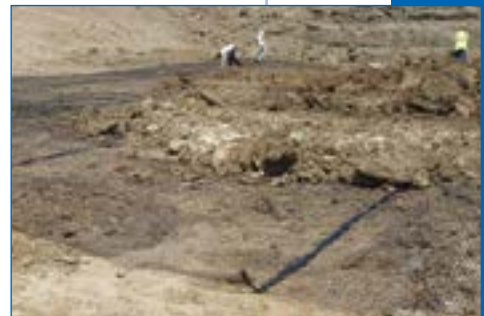
3 No overlapping of geogrid required.
