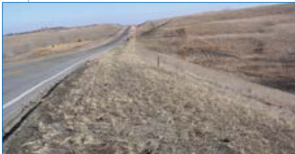
7 Highway restored to original condition.
