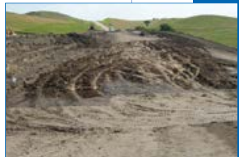
2 East slide construction.
