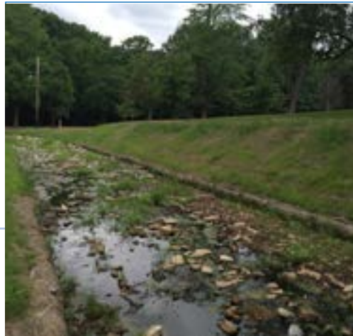
3 Coir fiber logs in place at Monroe Creek.
