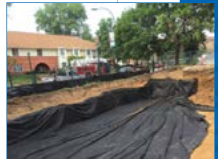
1 Site for BMP is excavated and soil compaction verified.
