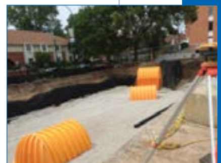
3 Arch chamber placement begins.
