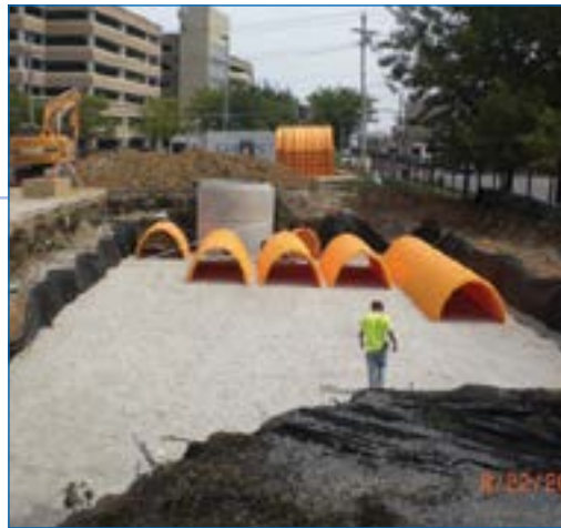
4 Subsequent rows of arch chambers are installed.
