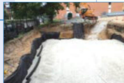
2 Placement of non-woven geotextile, clean aggregate and 6" N12 perforated underdrain pipe.
