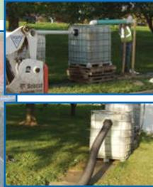
*From the collection pit to the treatment train. Gravity moves the water through the treatment train.*
