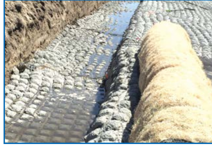
Flexamat in the anchor trench and ready to be deployed into the water.
