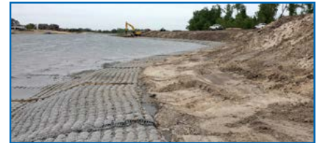
Flexamat in the anchor trench and ready to be deployed into the water.
