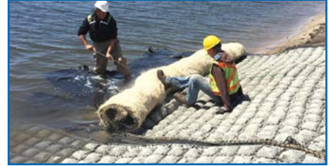
Flexamat in the anchor trench and ready to be deployed into the water.
