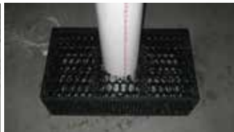
Figure 13: Place inspection port into underdrain module
