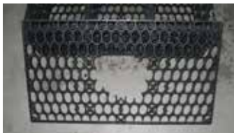
Figure 12: Cut 6" Hole into top panel of underdrain module to accommodate 6" pipe
