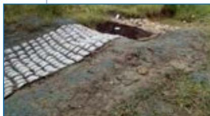
**6** After the rainevent, no erosion took place and the system was not inundated with sediment.
