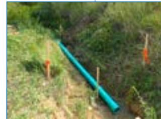
1 The outlet pipe was located with the proper 1% fall.
