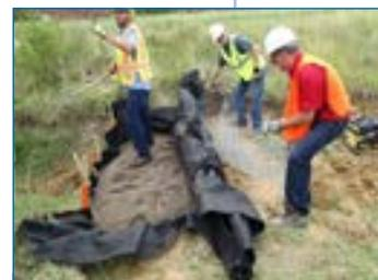
3 Installing the energy dissipating gabion weir.
