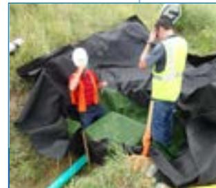
2 The underdrain system is installed and ready for pea gravel.
