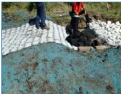
**4** Completed Focal Point with Spillway overflow, seeded berm and upstream energy disipation.
