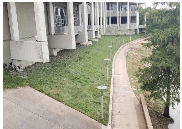
After Completed Installation
