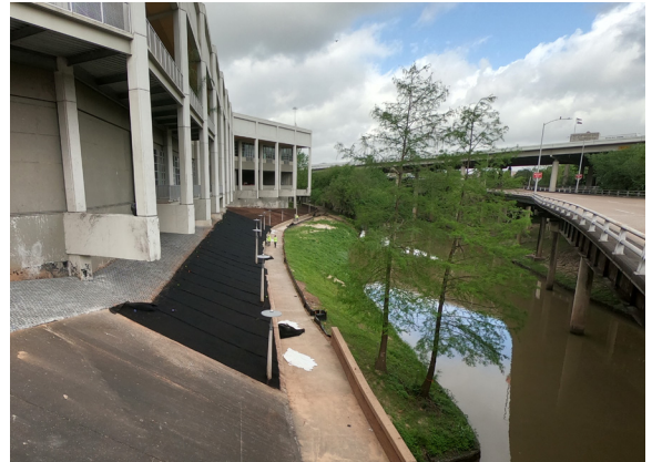
After Futerra® TRM Installation
