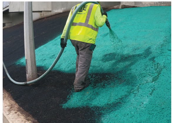
After Flexterra® Installation
