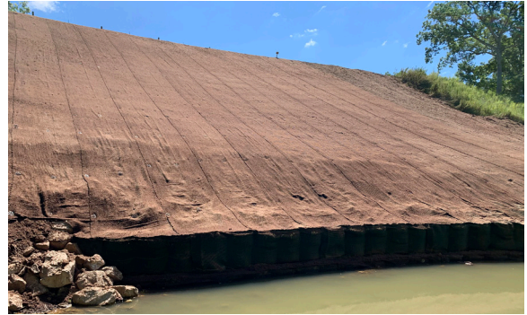
After ProGanics Installation
