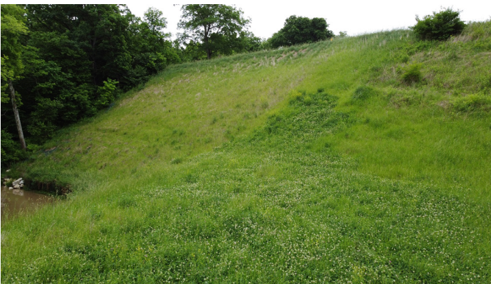
One year later the slope is fully vegetated and looks great.
