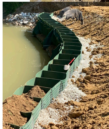
Installation of SCOURLOK complete. SCOURLOK filled with slope graded.
