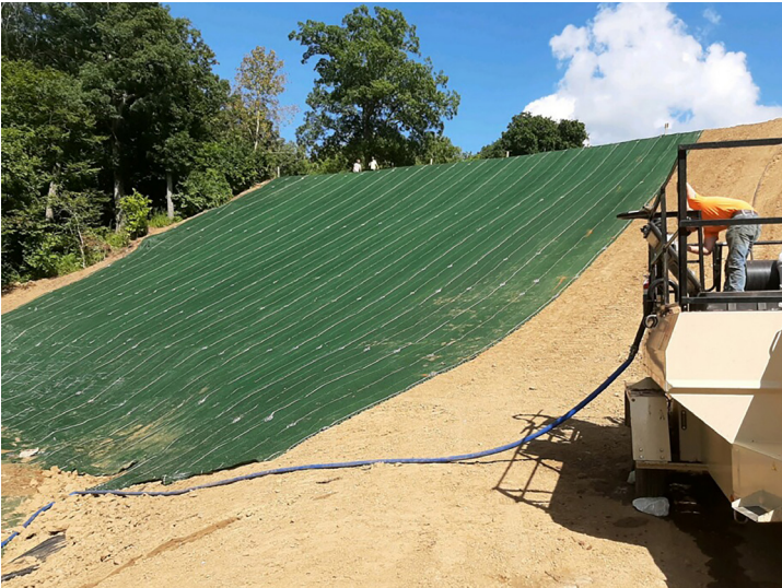
ARMORMAX Installation on Slope
