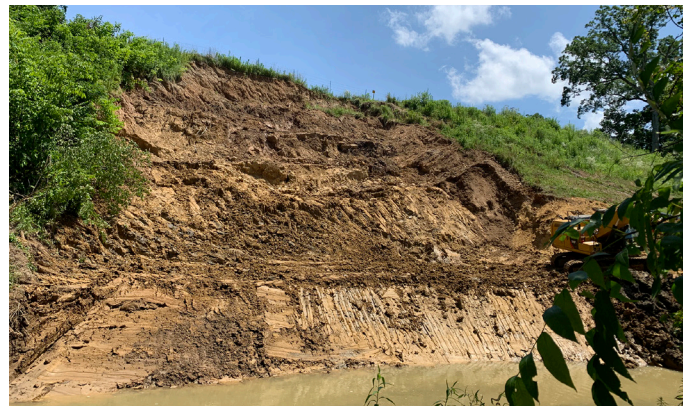
Removal of sloughed soil.
