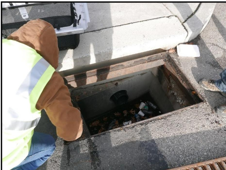
3. Using the catch basin frame clear opening length and width measurements from Step 2, adjust the sliding flanges such that they will securely rest on the grate frame. The inside flange to flange distance should be equal to the previously measured clear space for both length and width.
