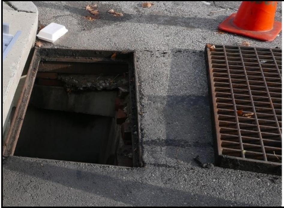
2. Measure and note the catch basin frame clear opening length and width. Remove any obstructions or debris that will interfere with the installed ScreenBox. If necessary, use a wire brush to remove caked on sediment from the grate support ledges.
